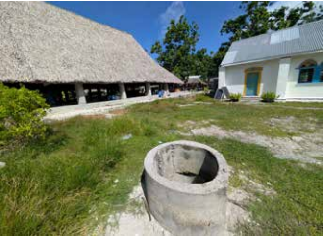
▲ A shallow water well in Abaiang. An MSF team is working to identify and rehabilitate wells that have been contaminated by salinity and coliform bacteria. © Pratistha Koirala/MSF
